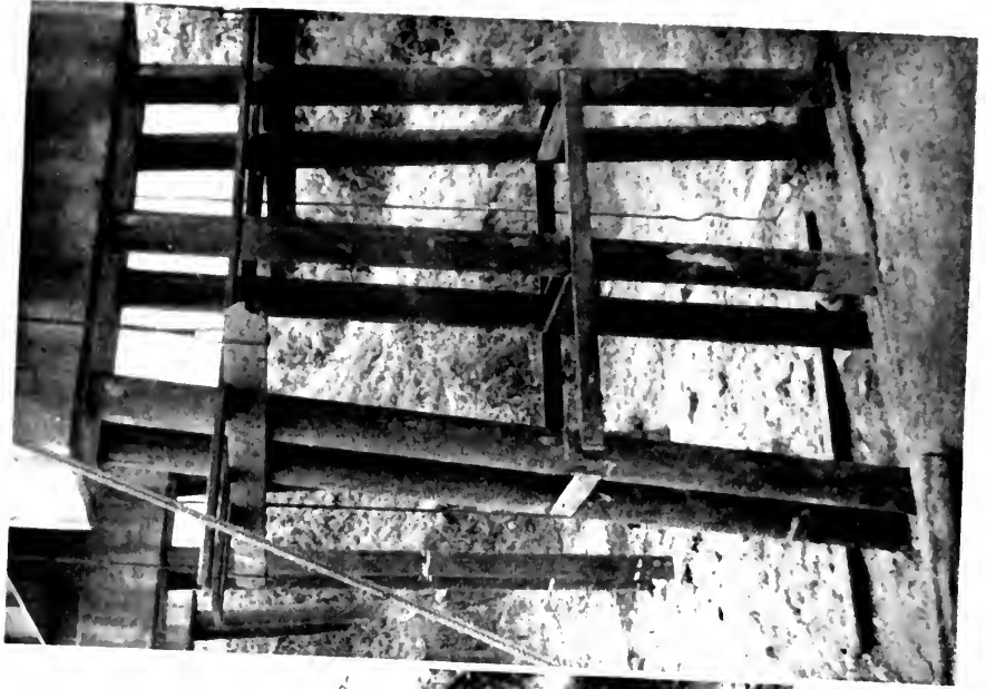
Fig. 3 (above)—View of pier 4, showing piles with timber bracing removed. Fig. 4 (right)—View of pier 3, showing new steel bracing welded to piles at 11 ft 1 in from bottom of concrete cap.
